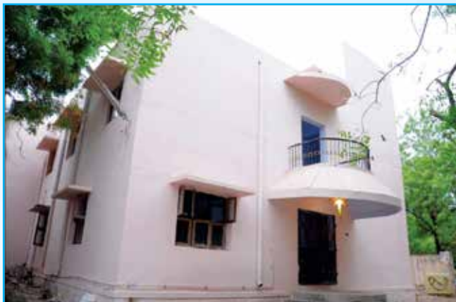
New First Floor in PG block of Girls hostel
